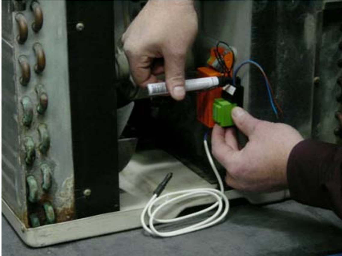
Marking the location of the transformer
